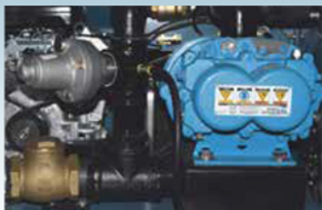
Positive Displacement Blower w/220 CFM @ 5PSI (Electric)
